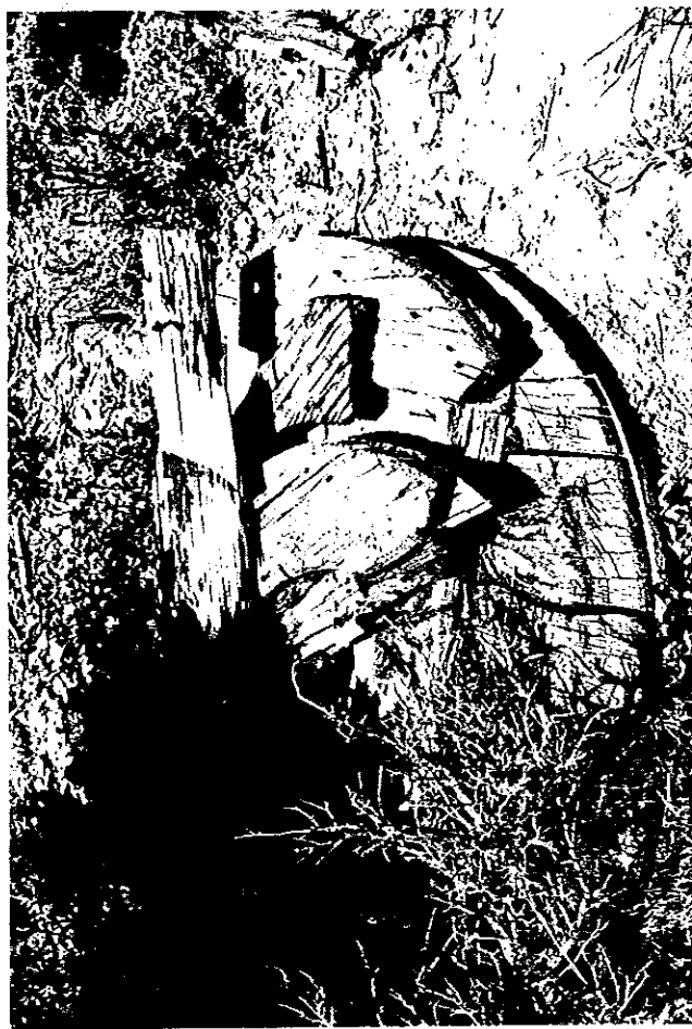
Figure 18. Crown Block Assembly
